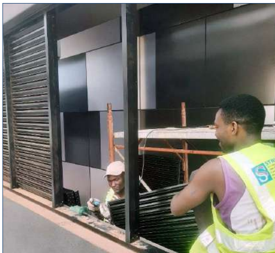
Installation of three sets of aluminium louvers
