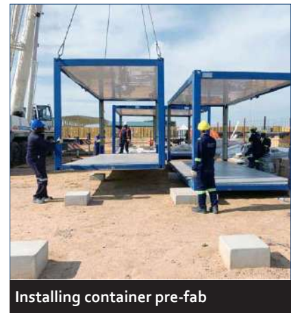
Walking slab installation/fitting
