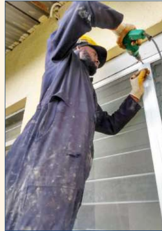
Fixing new external doors
