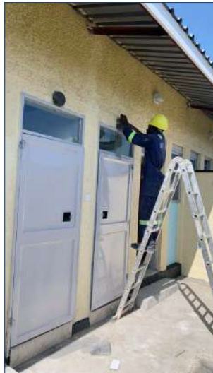
Fixing new external doors
