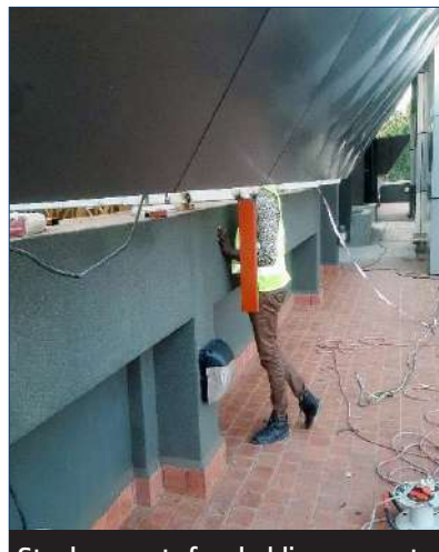
Steel supports for cladding supports being installed
