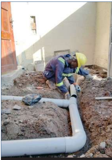
Repair of external drainage
