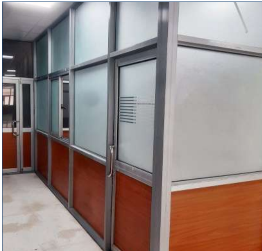
Fixed aluminium framing with MDF Board
