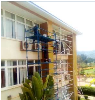
Erected scaffolds for painting of high points
