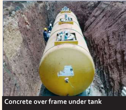
Backfilling with neutral coarse sand
